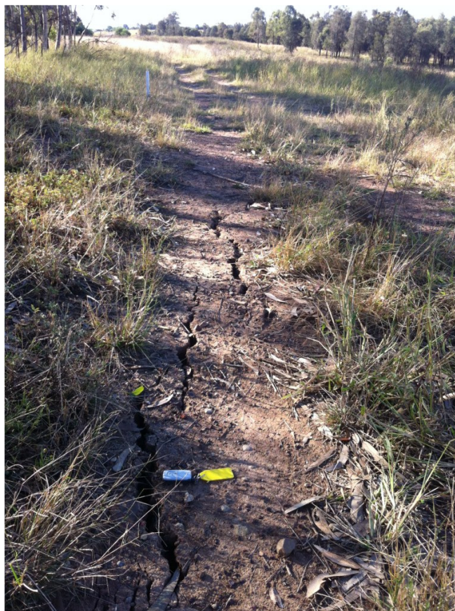
Figure 5: Surface crack along LW8 Maingate (3/05/12).
