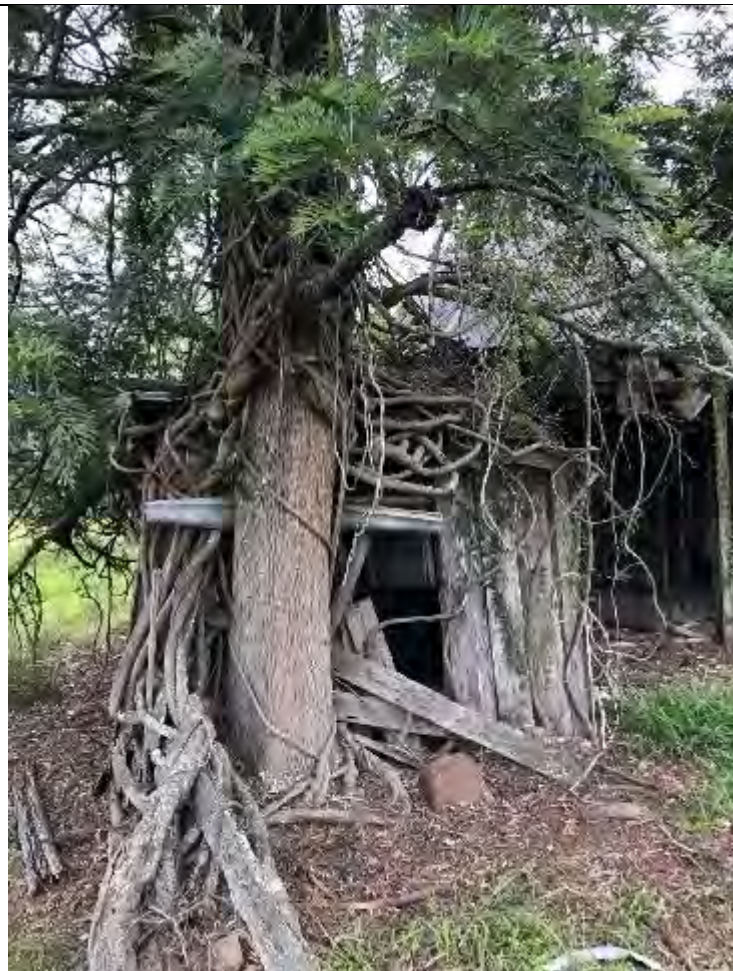
View of south-west corner from south: shows removal of vertical slabs from southern wall as well as some increase in vegetation growth.
