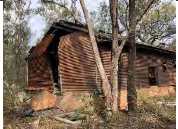
South-east elevation: evidence of increased bow to southern wall.
