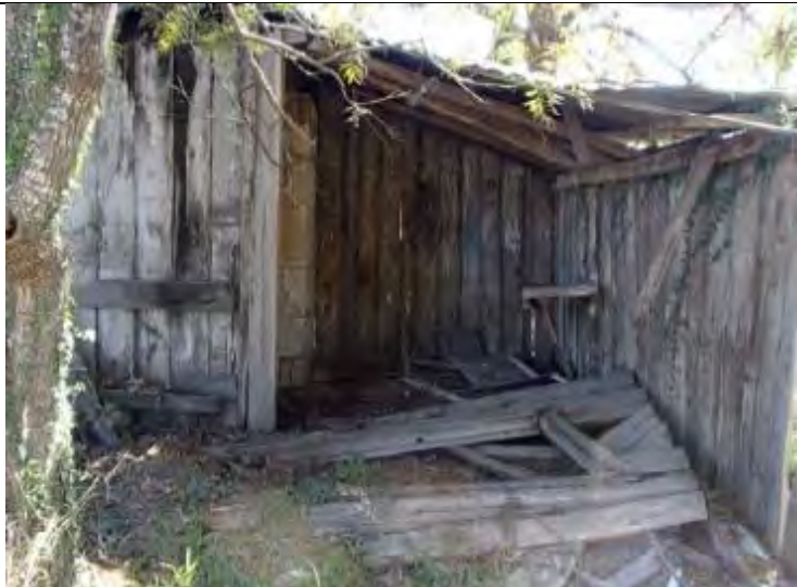
Northern elevation: further deterioration of weatherboard panelling.
