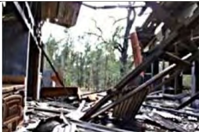
Showing interior of building, viewed from north-west corner: shows collapsed roofing members above open kitchen area and accumulation of debris.
