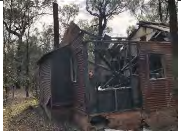
Detail of north-west elevation: shows increased collapse over open kitchen area, as well as new damage to brick foundation at north-west corner.
