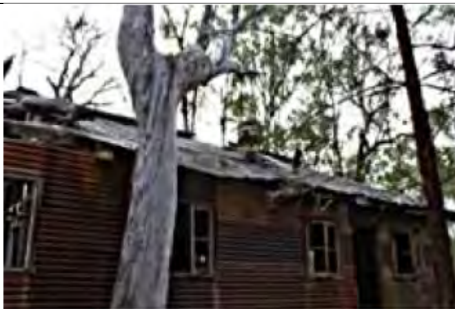
Showing cylindrical ventilator and damage to roof, view from west: shows significant roof damage from fallen dead tree, including to ventilator.
