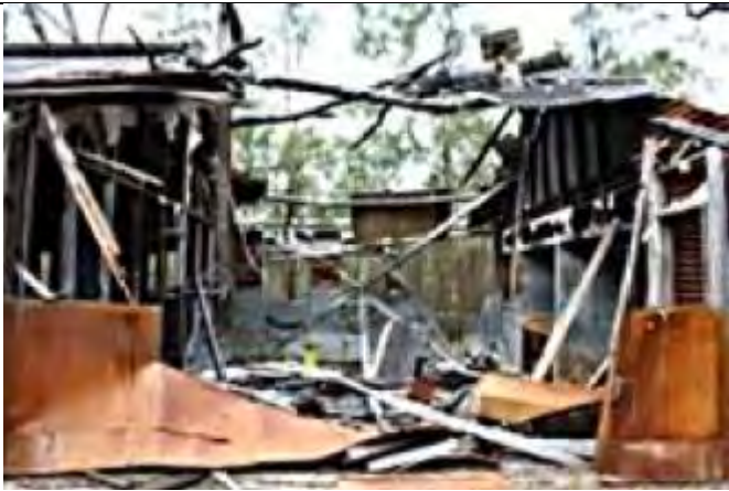
Showing interior damage at kitchen at north end of building: shows increased collapse over and accumulation of debris within open kitchen area. Note also severe lean to north wall.
