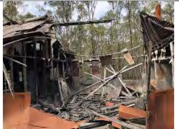
Showing interior damage at kitchen at north end of building: shows increased collapse over and accumulation of debris within open kitchen area. Note also severe lean to north wall.
