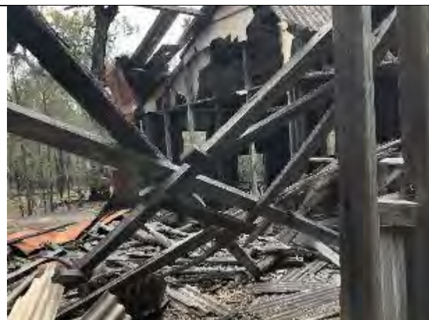
Showing interior of building, viewed from north-west corner: shows collapsed roofing members above open kitchen area and accumulation of debris.
