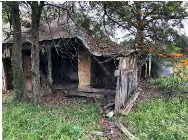
South-eastern corner: vertical slabs have been removed causing further collapse of roof.
