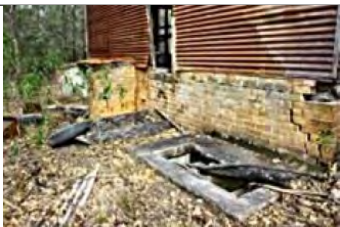
Grease trap at south end of building: shows bow to south wall.
