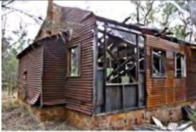
Detail of north-west elevation: shows increased collapse over open kitchen area, as well as new damage to brick foundation at north-west corner.
