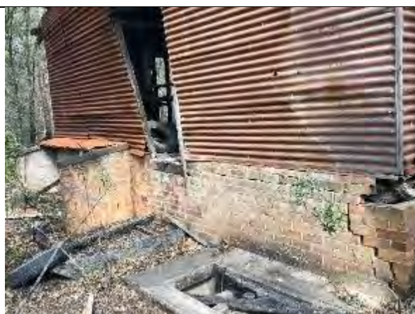
View to building interior from north-east: shows collapse of remnant roofing members above open kitchen area.
