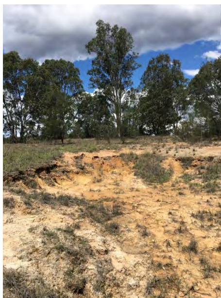
Plate 39 Erosion (top of right bank)
