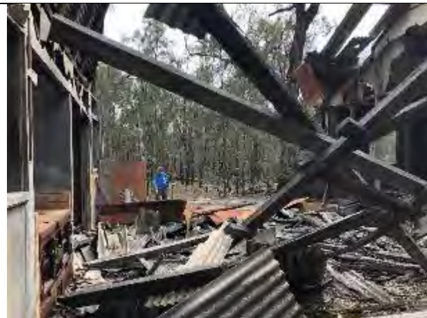
Showing interior of building, viewed from north-west corner: shows collapsed roofing members above open kitchen area and accumulation of debris.
