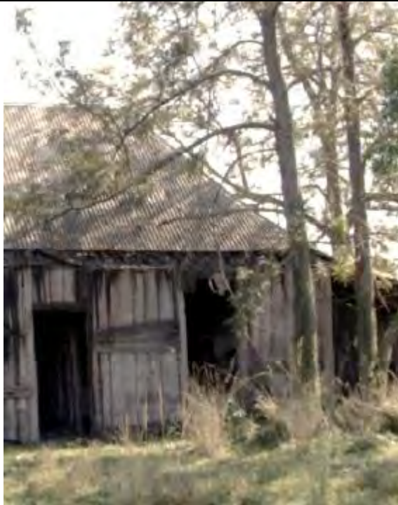
Southern elevation: vertical timber slabs have been removed from southern wall.
