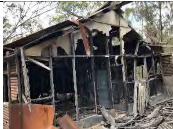
View to interior of south end of building, view from east: shows increased collapse over open kitchen area.
