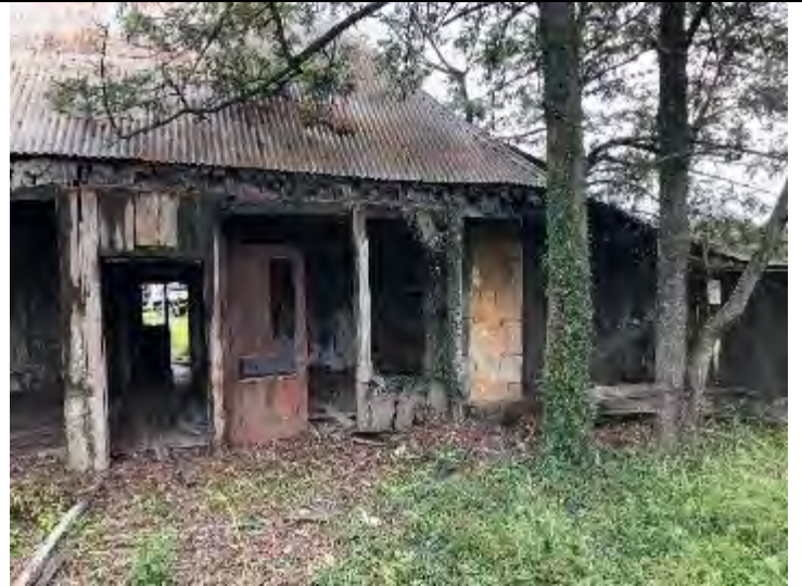
Southern elevation: vertical timber slabs have been removed from southern wall.
