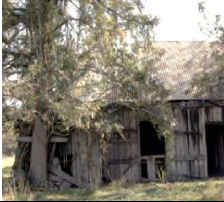
Southern elevation: vertical timber slabs have been removed from southern wall.
