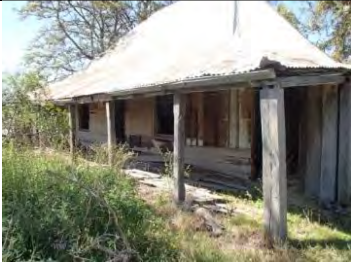
Northern elevation: slumping of verandah along edge beam.
