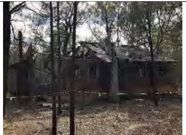
West elevation: shows deterioration of roofing members above open kitchen area and leaning north wall, and further collapse of asbestos roof due to fallen dead tree.
