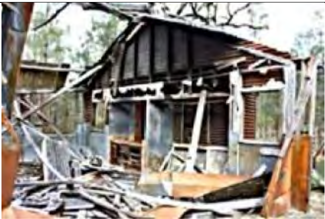
Showing interior damage at kitchen at north end of building: shows increased collapse over and accumulation of debris within open kitchen area. Note also severe lean to north wall.
