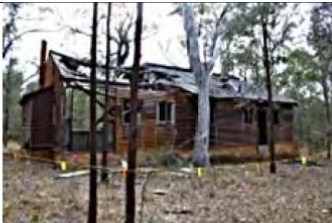
West elevation: shows deterioration of roofing members above open kitchen area and leaning north wall, and further collapse of asbestos roof due to fallen dead tree.
