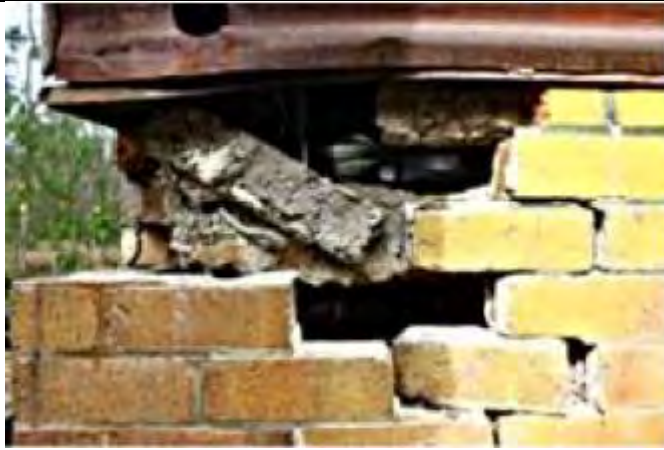
Detail of damaged brick foundation: some further collapse of concrete/cement above brick foundation.
