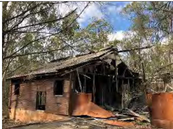
View to building interior from north-east: shows collapse of remnant roofing members above open kitchen area.
