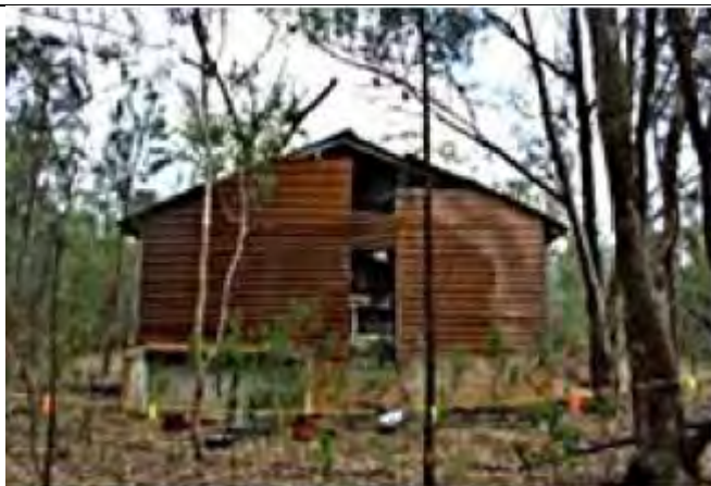
South elevation: evidence of increased bow to southern wall and missing panel above entry.
