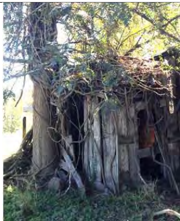
Looking towards south-west corner from east: no discernible change to tree impact, but note missing vertical slabs from southern wall.
