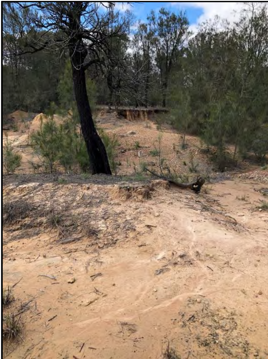
MTW-655 located around and across eroding gully
