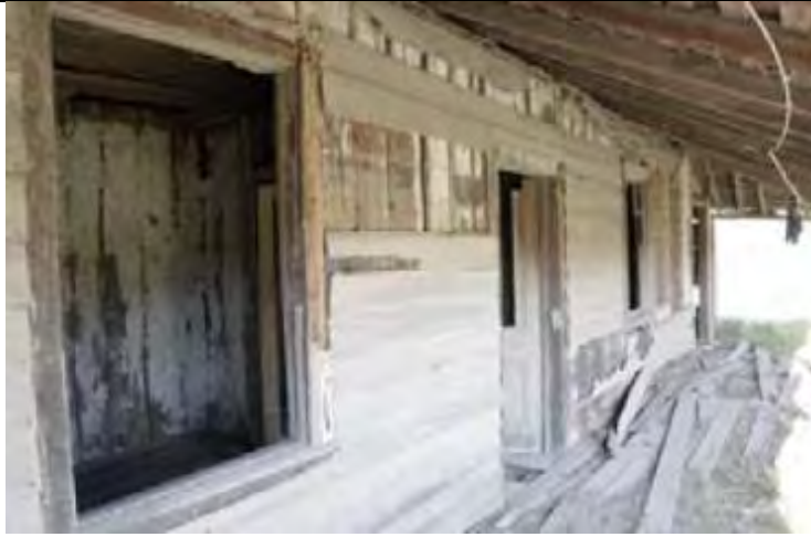
Northern elevation: further deterioration of weatherboard panelling.
