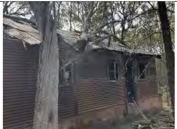
Showing cylindrical ventilator and damage to roof, view from west: shows significant roof damage from fallen dead tree, including to ventilator.
