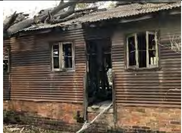
Windows and entry at west elevation: shows large trunk/branch portions of tree collapsed on roof, which has destroyed roof ventilator.
