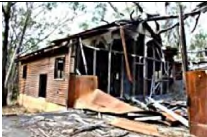
View to building interior from north-east: shows collapse of remnant roofing members above open kitchen area.
