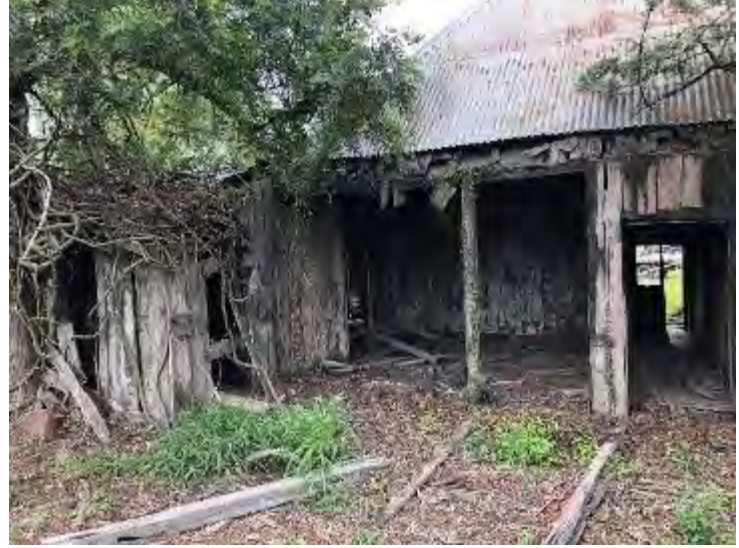
Southern elevation: vertical timber slabs have been removed from southern wall.
