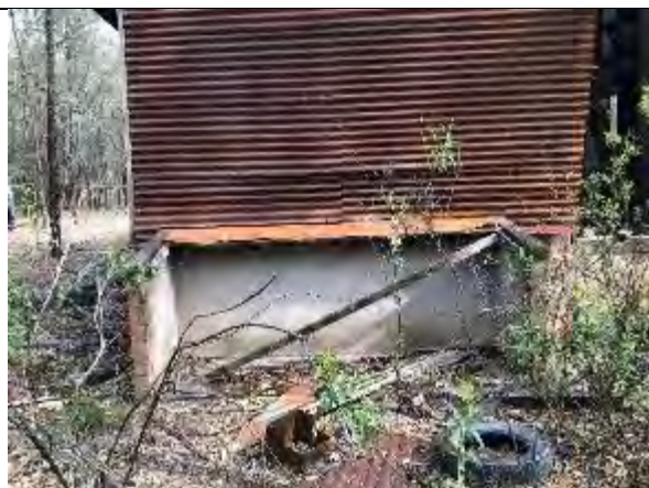
Storage area at south end of building: further slight collapse of storage area.
