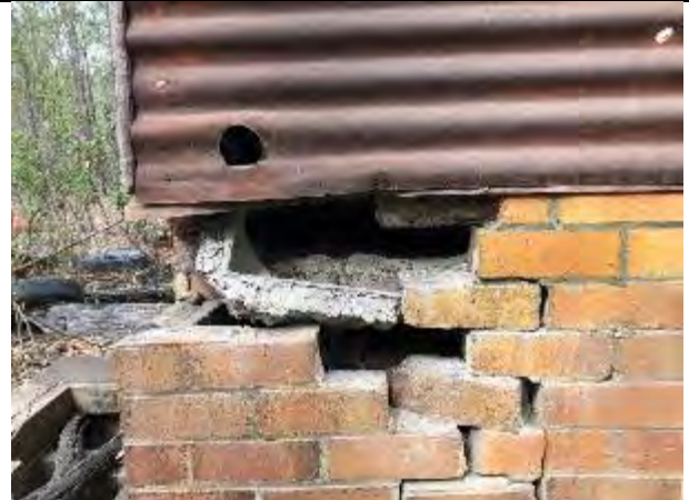
Detail of damaged brick foundation: some further collapse of concrete/cement above brick foundation.
