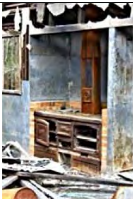
Showing stove at kitchen at north end: note the remaining two stove doors have become unhinged and build up of debris from collapsed roof.
