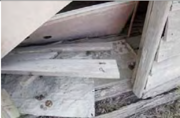
Southern elevation: vertical timber slabs have been removed from southern wall.
