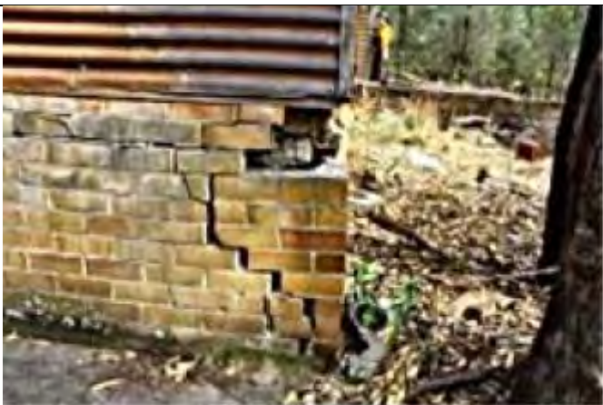
Damaged brick foundation at south-east corner: no discernible increase to cracked brick foundation.
