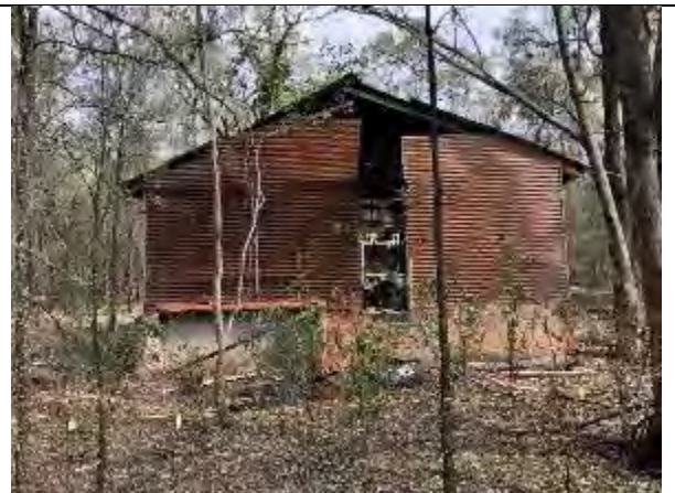
South elevation: evidence of increased bow to southern wall and missing panel above entry.
