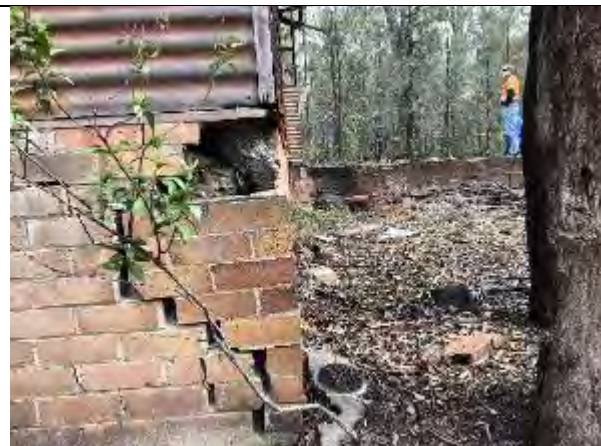
Damaged brick foundation at south-east corner: no discernible increase to cracked brick foundation.
