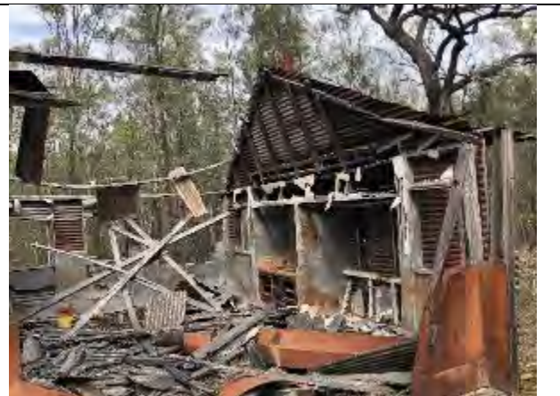
Showing interior damage at kitchen at north end of building: shows increased collapse over and accumulation of debris within open kitchen area. Note also severe lean to north wall.
