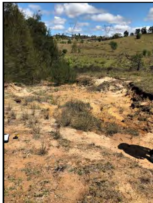
Erosion at MTW-639
