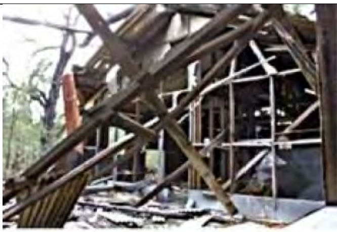
Showing interior of building, viewed from north-west corner: shows collapsed roofing members above open kitchen area and accumulation of debris.
