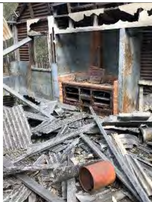
Showing stove at kitchen at north end: note the remaining two stove doors have become unhinged and build up of debris from collapsed roof.
