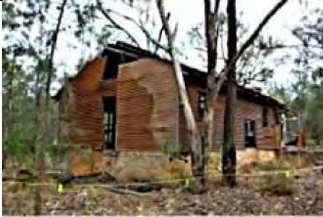
South-east elevation: evidence of increased bow to southern wall.
