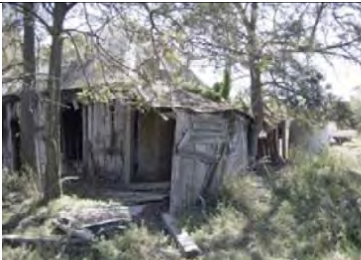
South-eastern corner: vertical slabs have been removed causing further collapse of roof.
