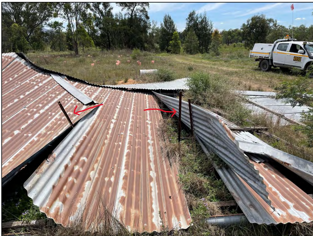
Star pickets indicate location of artefacts at MTW-668 underneath collapsed shed
