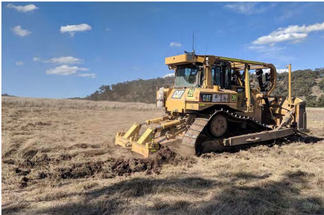
FIGURE 87: RIPPING BEING UNDERTAKEN IN THE GOULBURN RIVER BIODIVERSITY AREA
