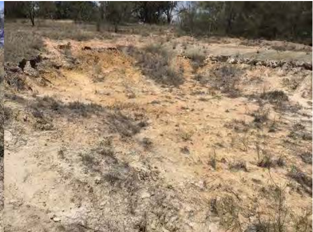
Plate 37 Erosion (top of right bank)
