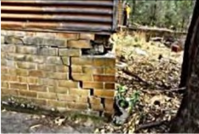
Damaged brick foundation at south-east corner 2012-18: no discernible increase to cracked brick foundation. 2018-20: further cracking of foundation (to left of shot) and some slumping of corner bricks.
