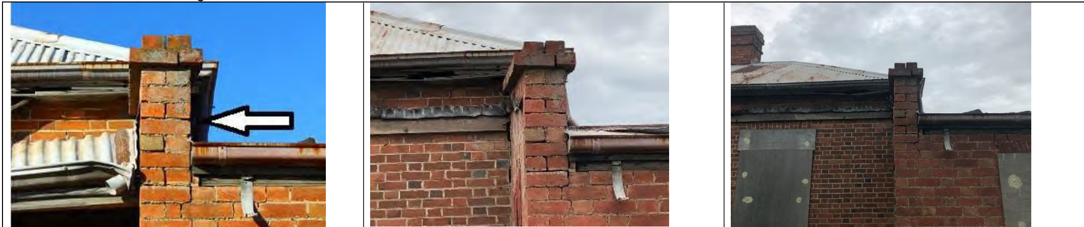
View of south-east of building (focus on top of wall) 2015-8: no discernible change 2018-20: no discernible change
