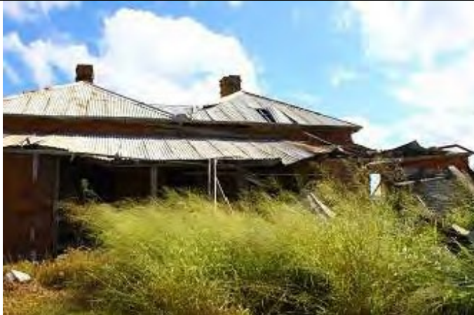
View of rear of building (focus on guttering) 2015-8: main roof holes repaired but northern section of skillion roof collapsed and guttering unchanged 2018-20: no discernible change, however vegetation regrowth evident
