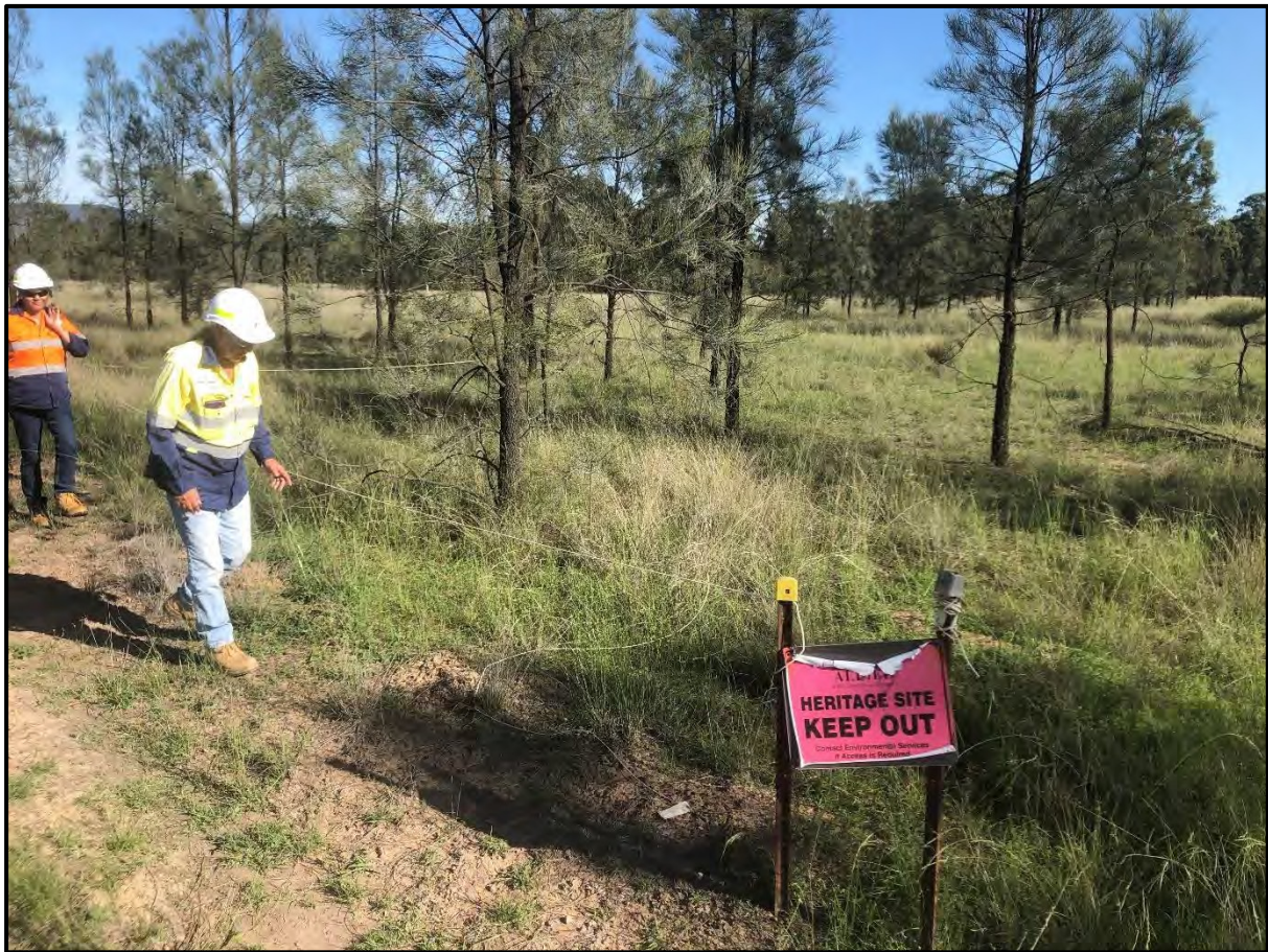
Example of dilapidated barricading
