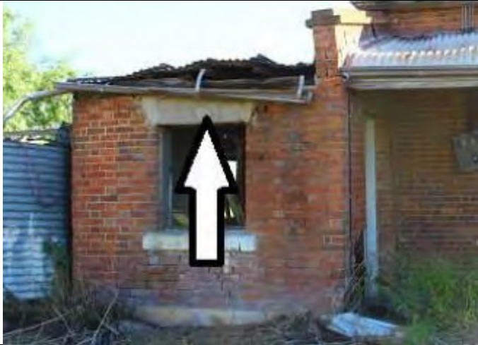
View of north-east of building (focus on skillion roof) 2015-8: roof framing, sheeting and guttering has collapsed 2018-20: no discernible change
