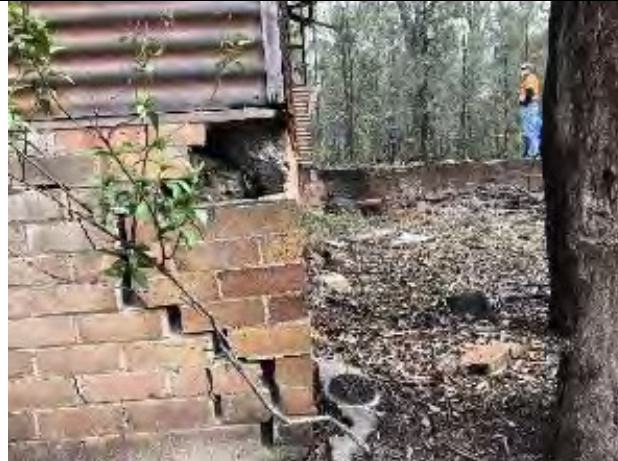
Damaged brick foundation at south-east corner 2012-18: no discernible increase to cracked brick foundation. 2018-20: further cracking of foundation (to left of shot) and some slumping of corner bricks.
