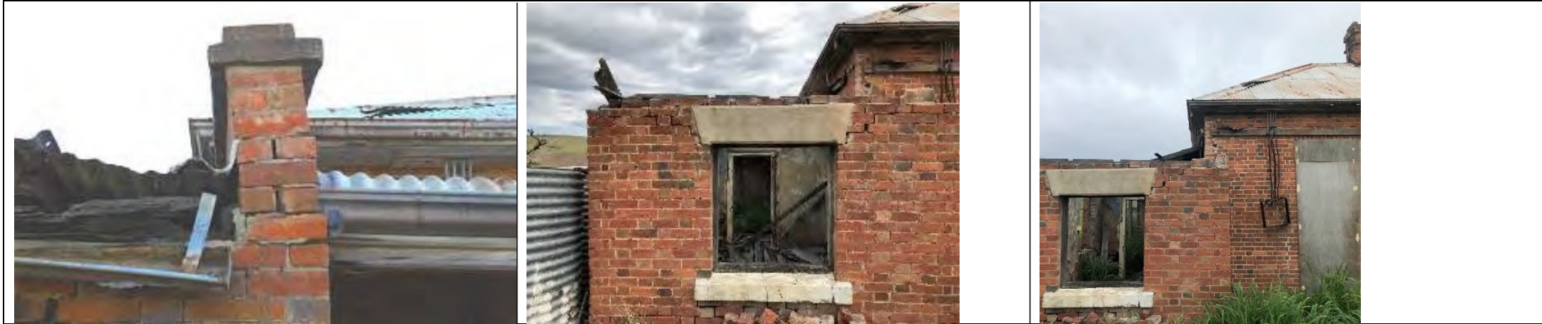
View of north-east of building (focus on top of wall) 2015-8: wall element has collapsed bricks stacked under window) 2018-20: no discernible change
