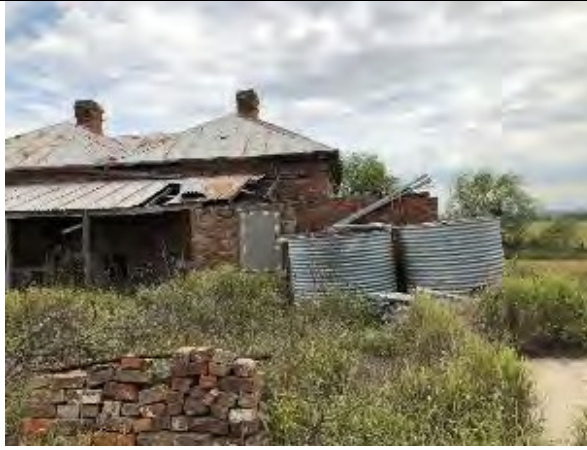
View of rear of building (focus on guttering) 2015-8: main roof holes repaired but northern section of skillion roof collapsed and guttering unchanged 2018-20: no discernible change, however vegetation regrowth evident
