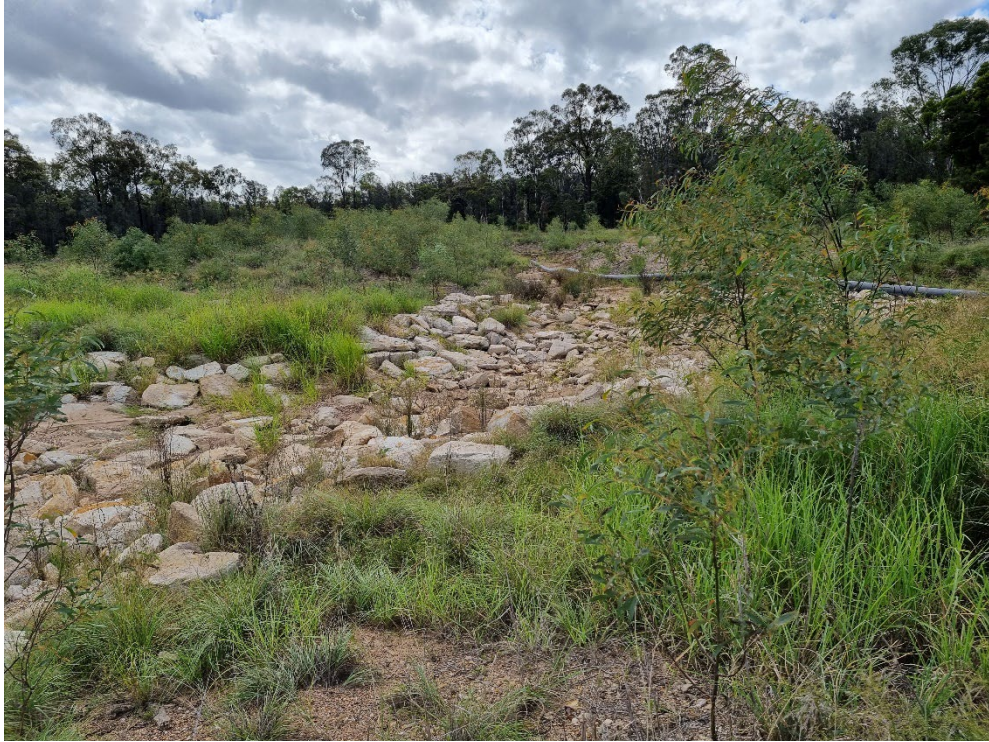
Photograph 5 - Stabilised Drain
