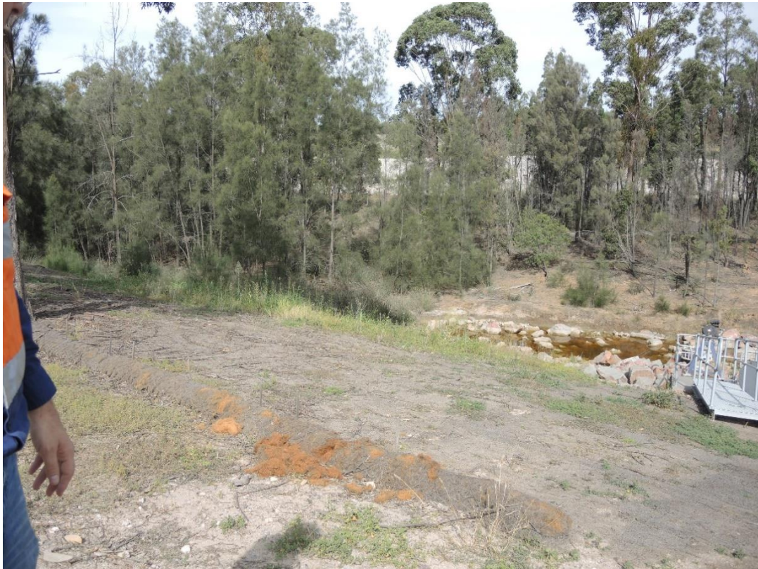
Plate 13 Creek stability improvement works at Dam 9s HRSTS discharge location
