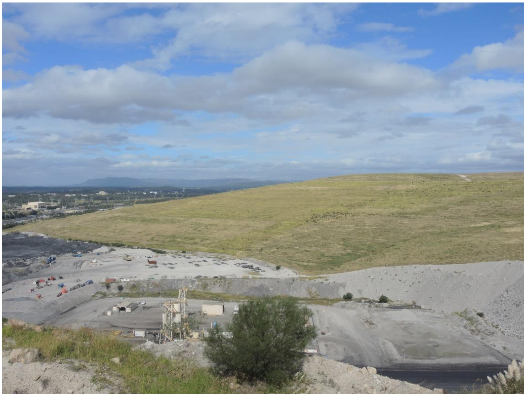
Plate 20 Area of rehabilitation adjacent to the explosive's facility
