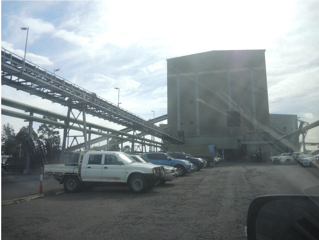
Plate 3 Mount Thorley CHPP and CHPP mid sized circuit
