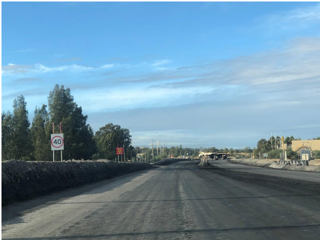
Plate 6 Warkworth haul roads
