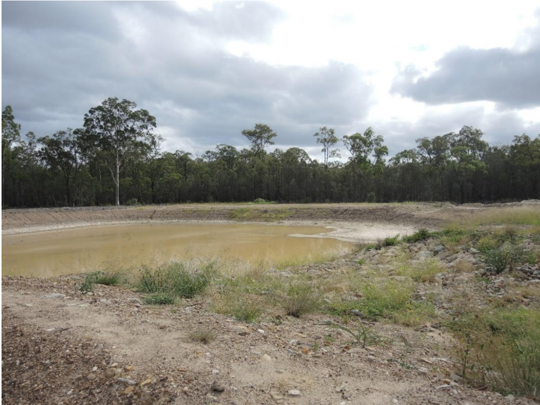
Plate 11 Western sediment dams constructed in 2018
