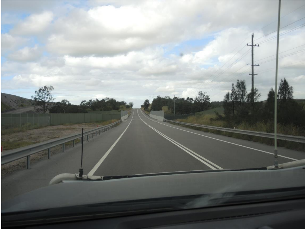
Plate 17 Putty Road third underpass constructed during the IEA period
