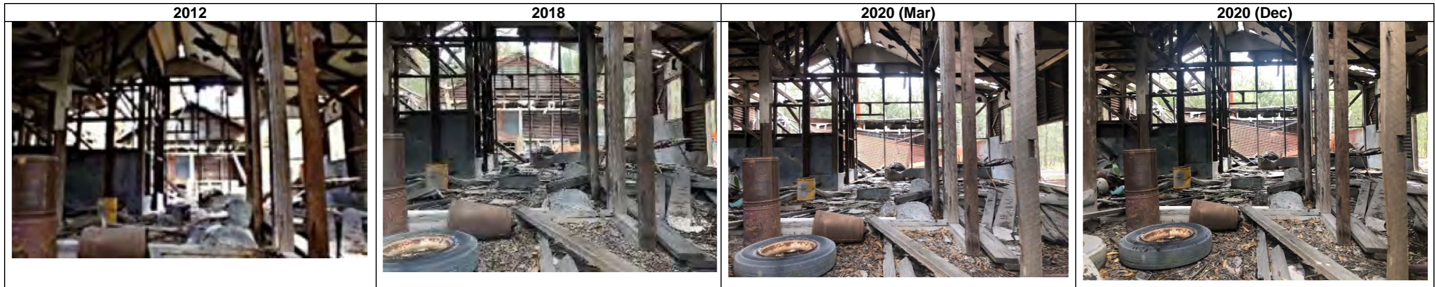
View to interior of building, looking north from south entry
