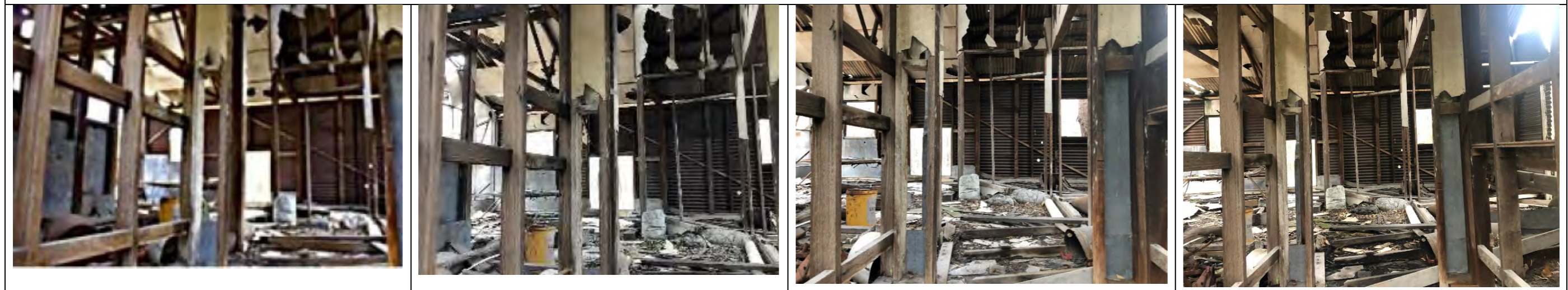
View to interior of building from entry at west
