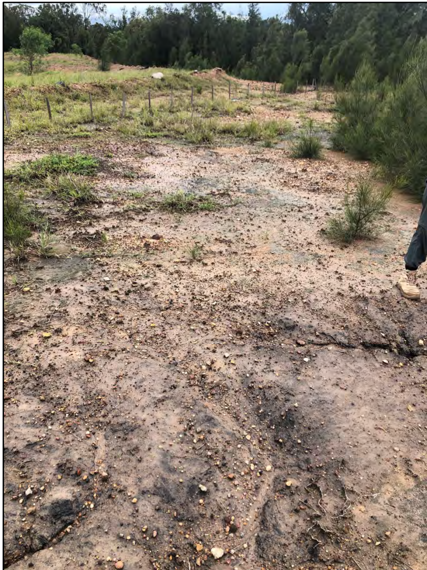
Sheet wash erosion at MTW-548
