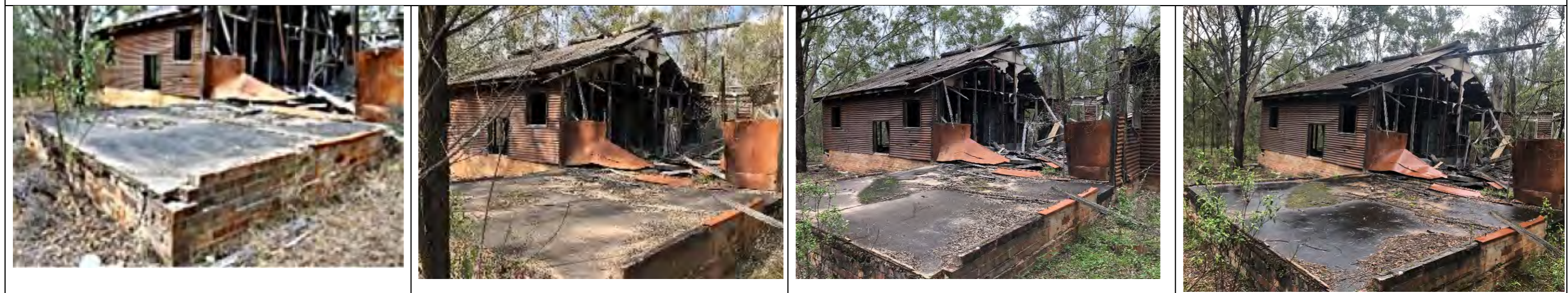
Concrete and brick foundation at east side of building 2012-18: difficult to discern change. 2018-20 (Mar): no discernible change. Mar 2020 – Dec 2020: no discernible change.
