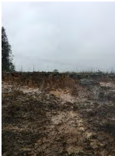
Plate 9 Erosion (top of right bank)
